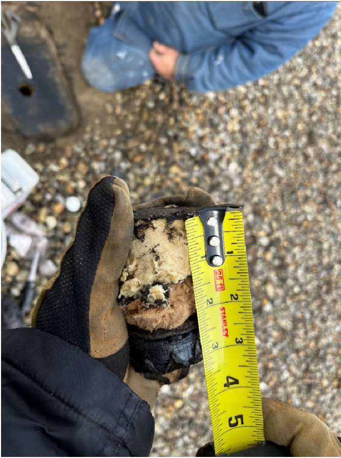
Beu Health Center – Core at roof drain
