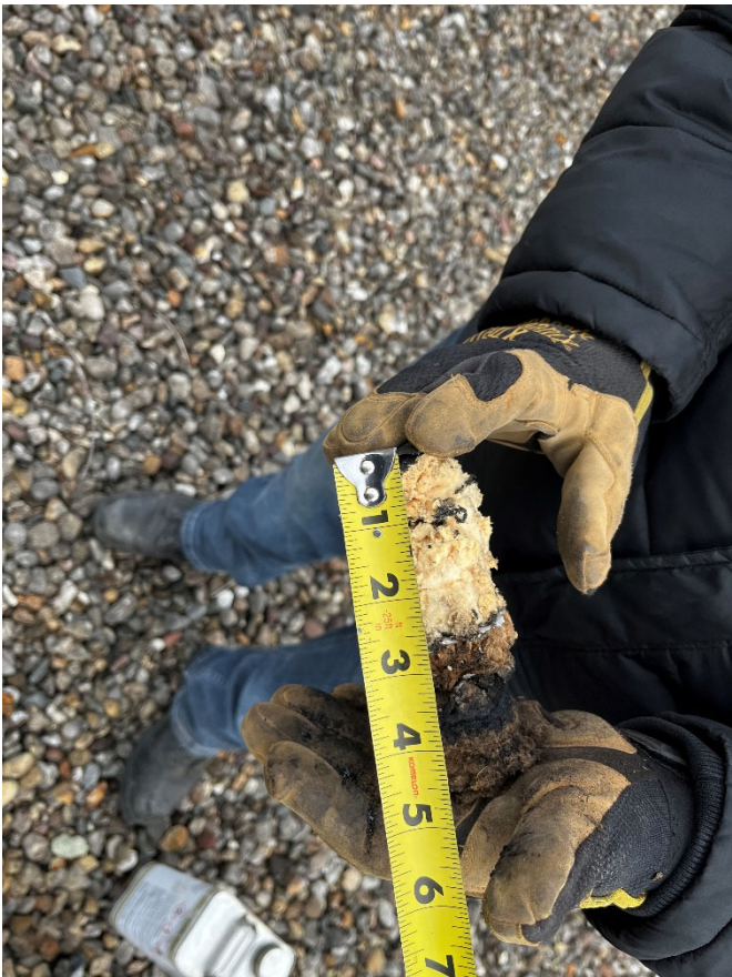
Beu Health Center – Core at roof edge
